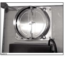
2. Remove protective plastic film on the lower flue and install it over the hood.
